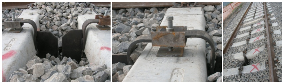
Figure 8: Shovels installed on the sleepers.
