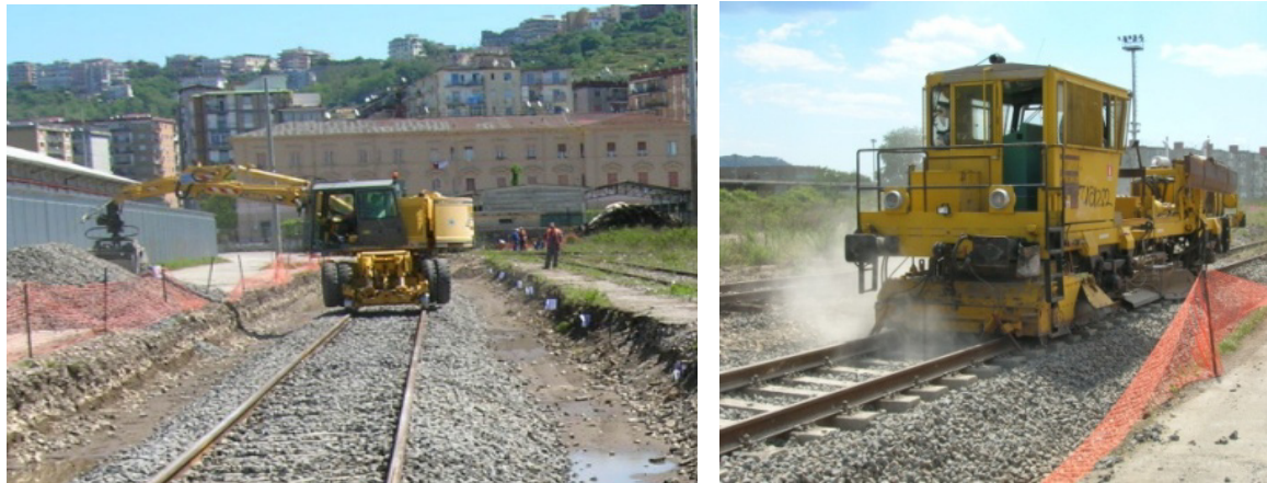
Figure 6: Deposition of the ballast (left) and removing of the excess (right).
