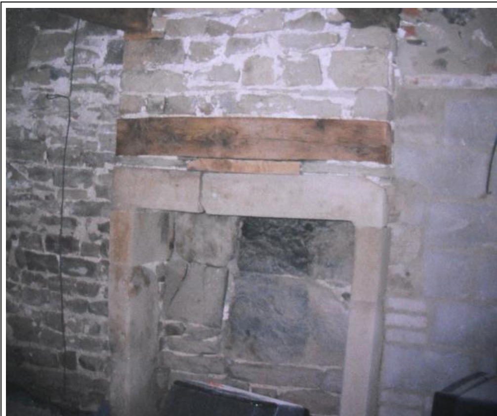
Figure 12 – Fireplace in which ILKLEY 1 was found. (Photograph by Kate Armitage)
