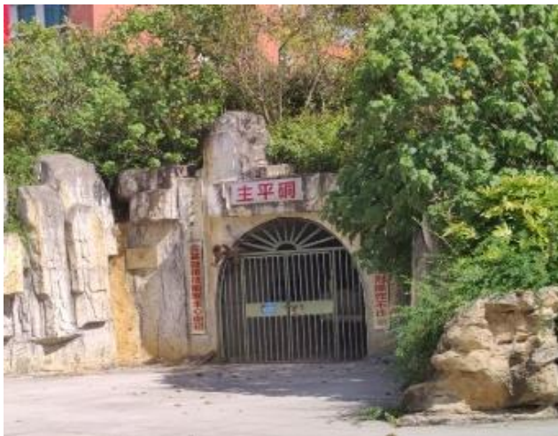
9 10 (c) Main tunnel
