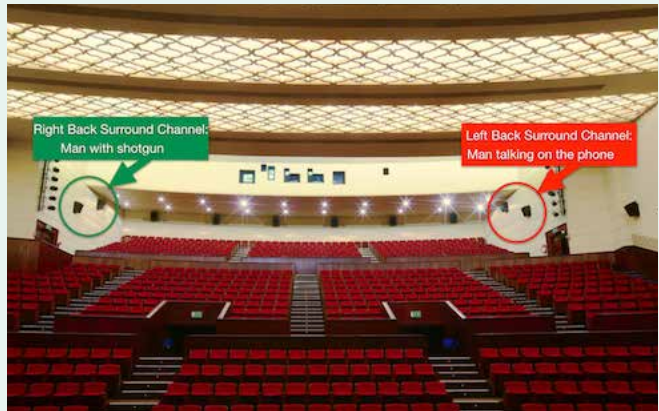
The channel placement in the cinema room - MINI Case Study
