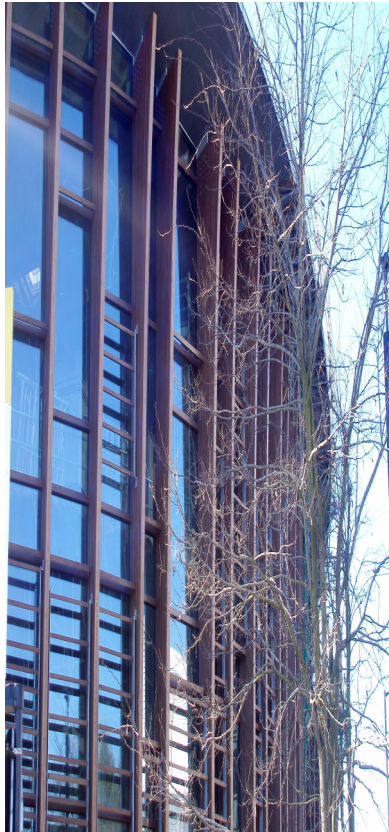
View of external walls showing tree-like columns and curved roof structure.
