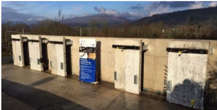
216 217 Figure 3 Self-healing concrete wall panels constructed within the EPSRC and industry funded 218 Materials for Life (M4L) project [35].
