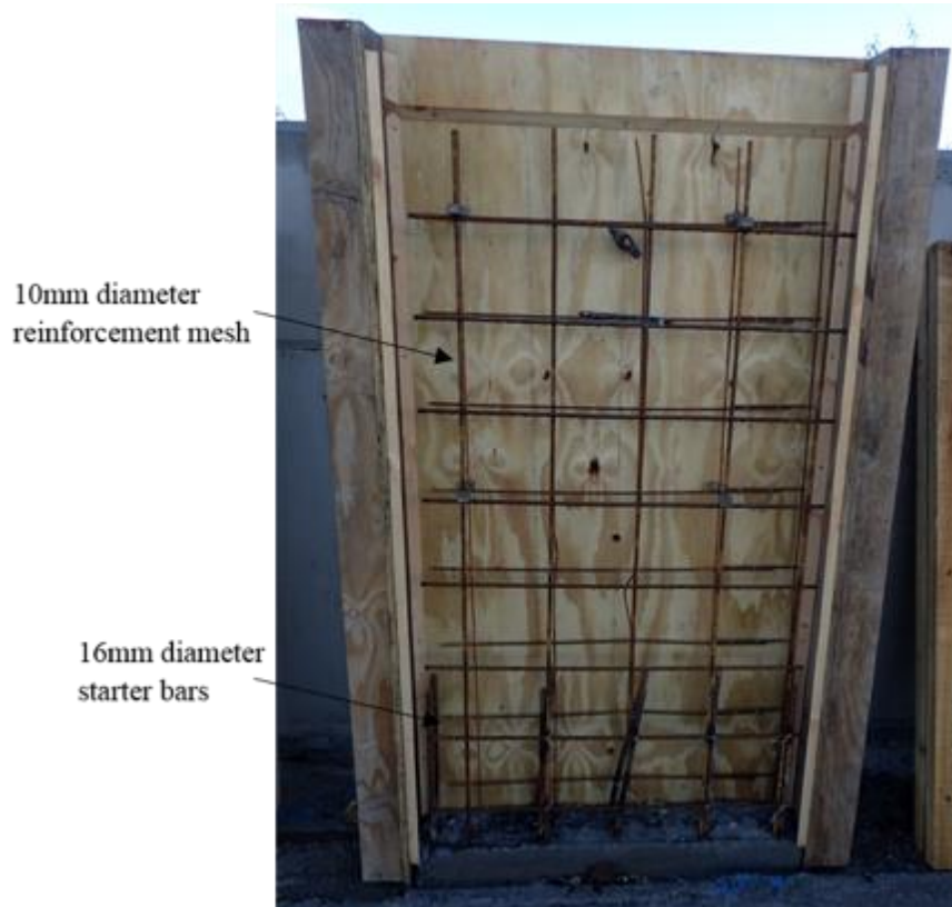
272 273 Figure 5 Wall panel reinforcement design to ensure cracking at ~500mm from the base of the wall 274 panel.
