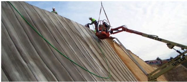
Fig.1 Concrete Canvas applied for slope protection
