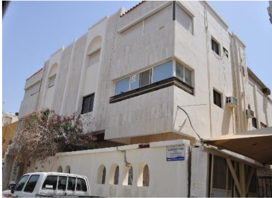
Figure 8-4 Covered balconies in Jeddah
