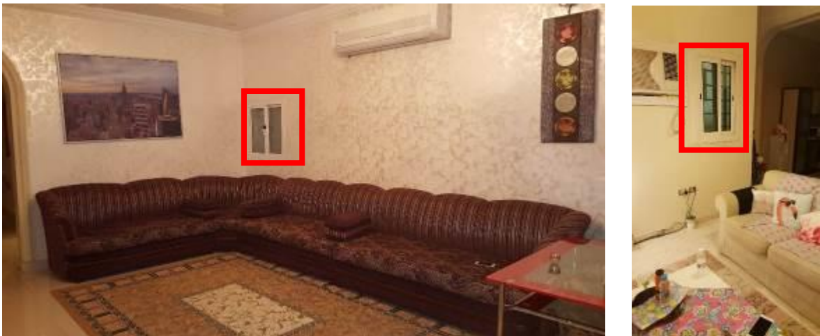
Figure 6-2 Light well windows in the living space. Left: third floor. Right: first floor
