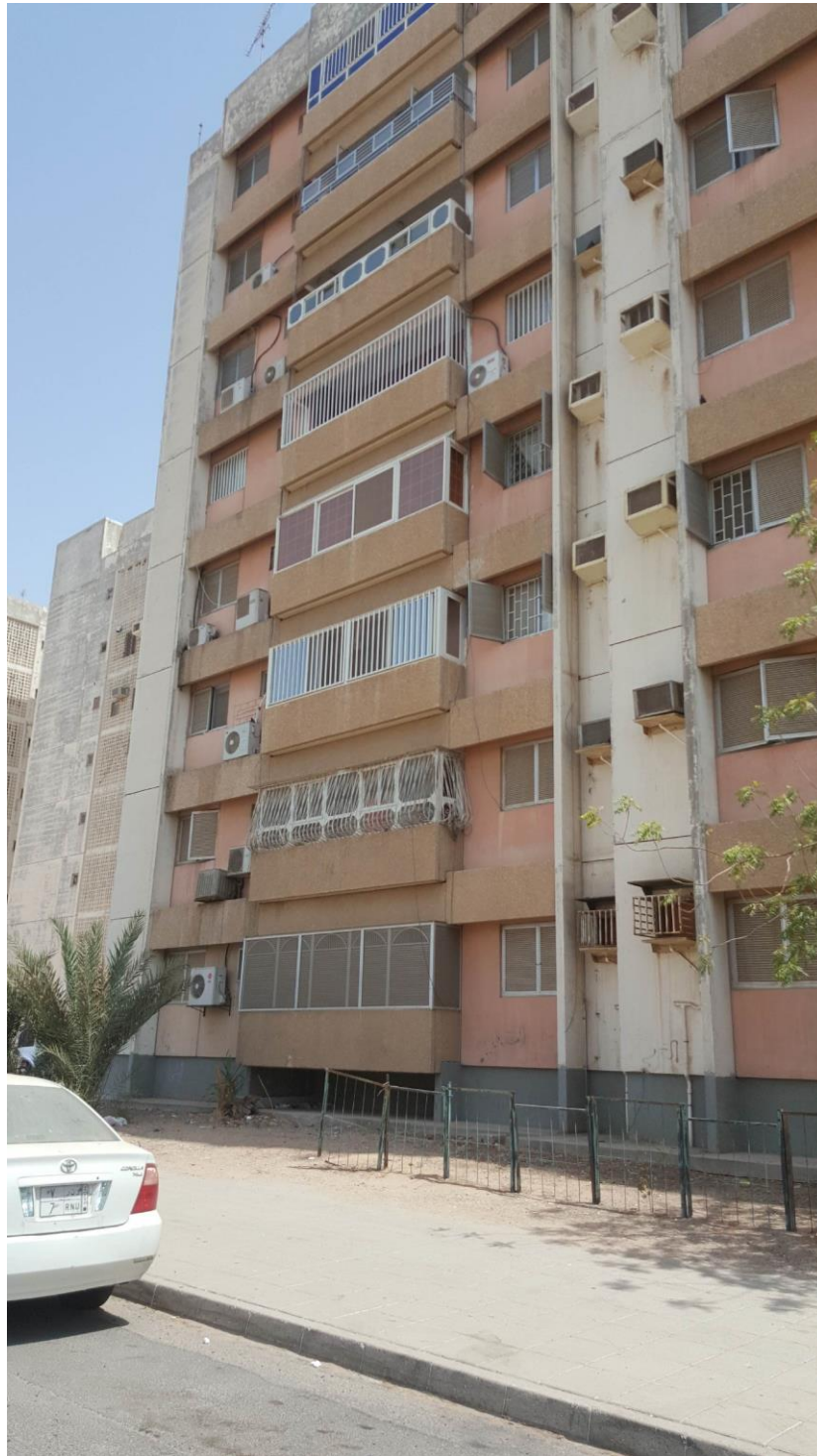
Figure 2-6 Privacy problems with balconies and windows in Jeddah
