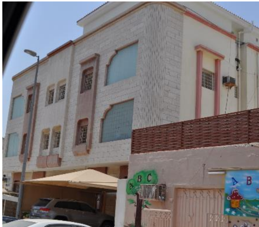
Figure 8-3 Covered balcony with black tinted glass in Jeddah
