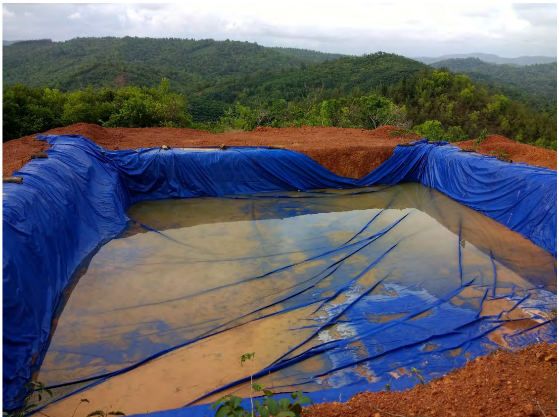
Figure 5.22: An overhead water tank under construction on a hilltop.
