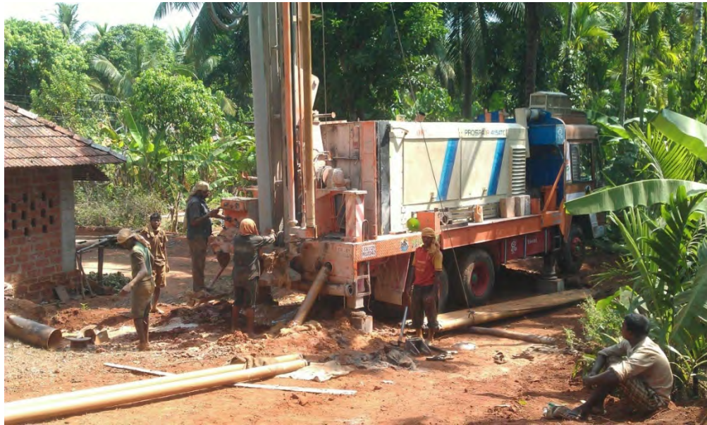
Figure 7.21: A borewell being constructed in Manila village in 2013 CE.
