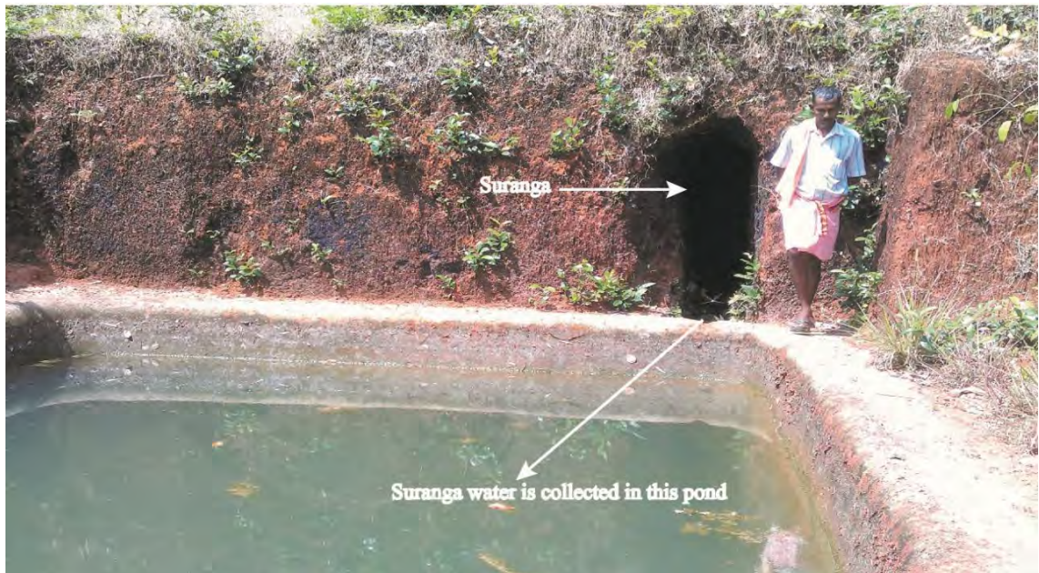
Figure 5.18: Earthen pond to collect suranga water.
