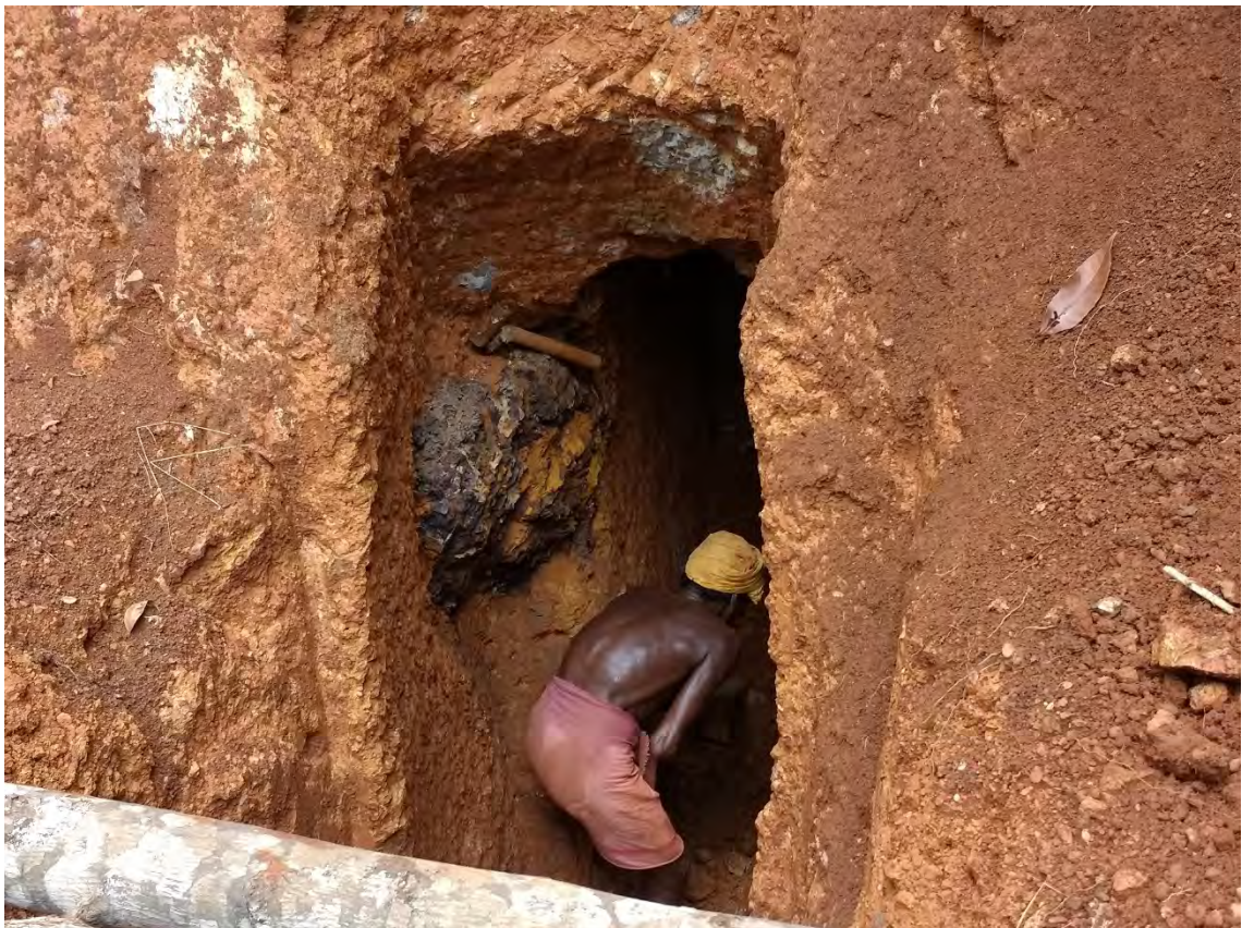
Figure 5.5: A suranga worker during the excavation of a suranga .
