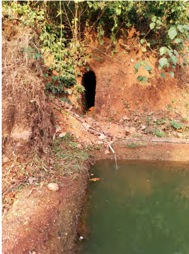
Figure 5.19: Earthen pond to collect the suranga water through a pipe.
