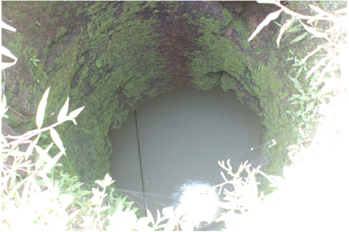
Figure 5.39: Looking down an airshaft with a submerged suranga .
