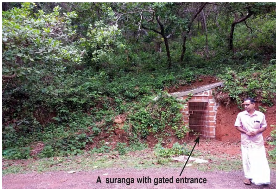
Figure 5.17: A drinking water suranga covered with a metal gate.
