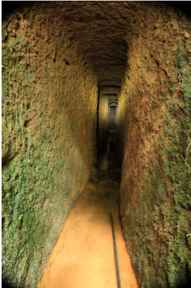
Figure 5.15: Water from a suranga being transported with a pipe.
