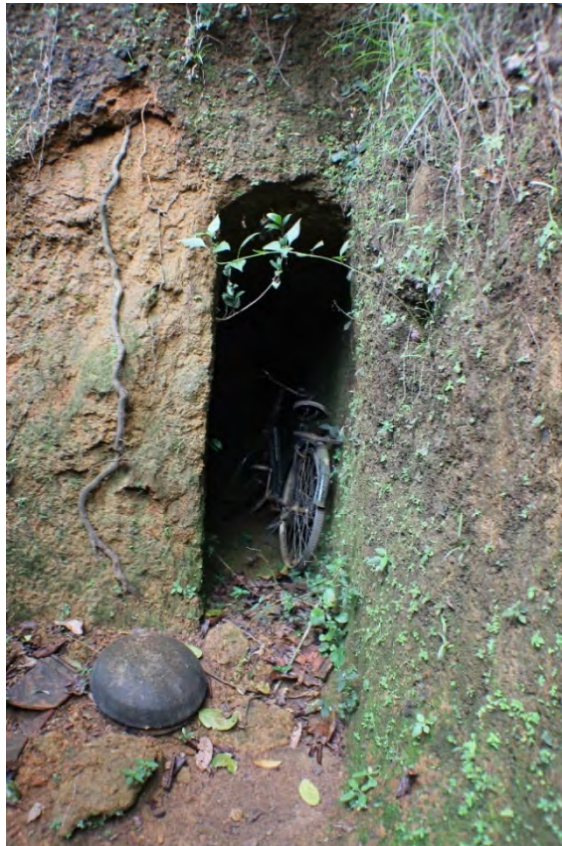
Figure 5.25: A dry suranga being used for storage.
