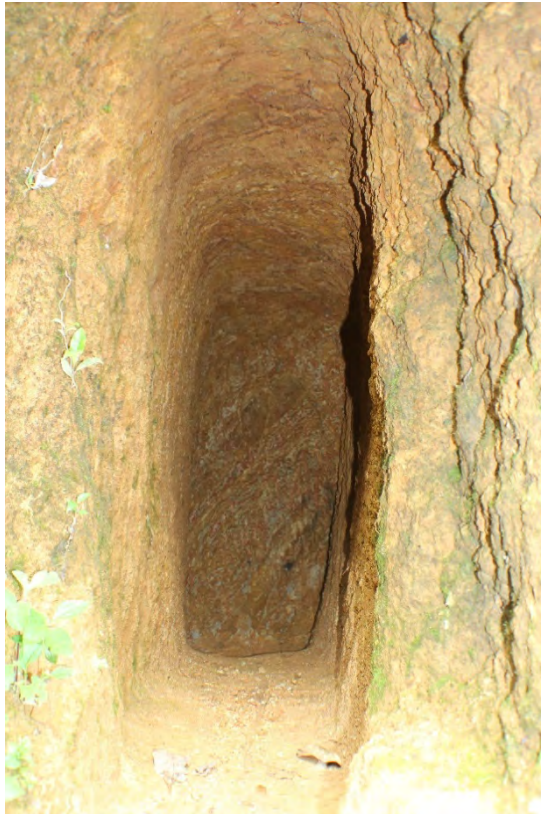
Figure 7.24: An abandoned small length suranga with hard rock dead-end.
