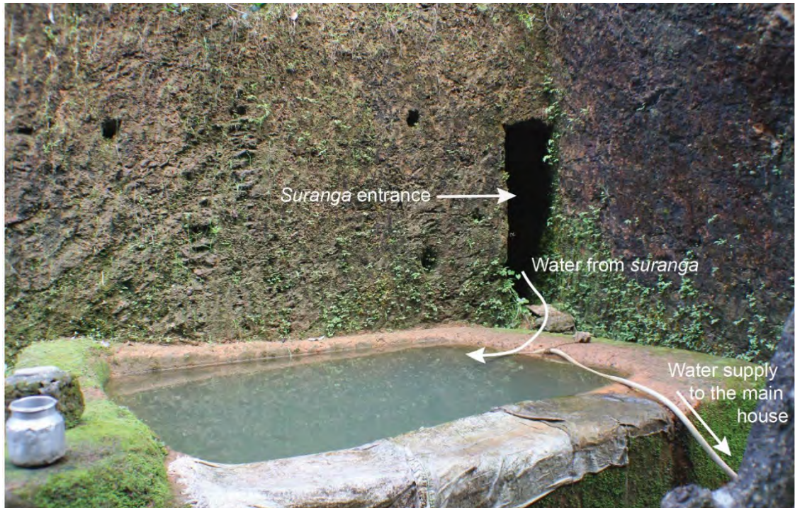
Figure 5.28: Drinking water supply with a pipe from an elevated suranga .
