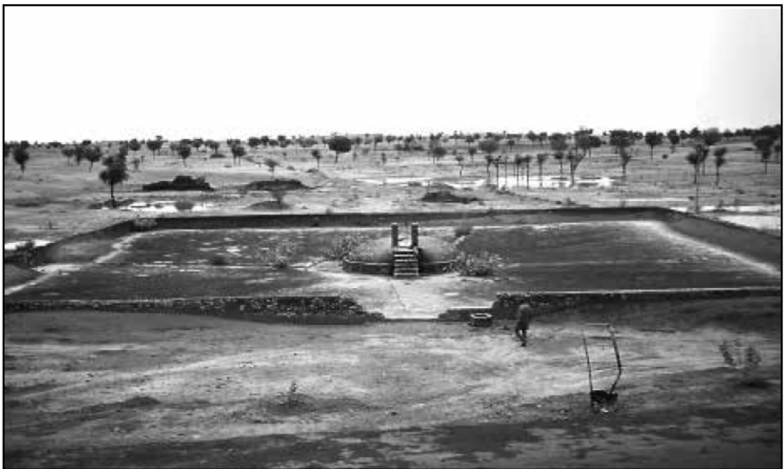
Figure 1.4: Picture of an underground rectangular, covered tank in the Thar Desert, with access at the centre through steps, and water is lifted manually through a rope and a bucket (Image source: Mishra, 2012).
