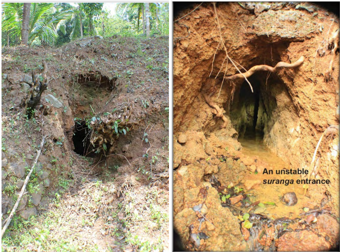
Figure 5.46: Two structurally unsafe suranga .
