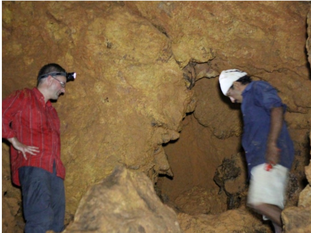
Figure 5.43: Inside view of a natural cavity caused by soil piping.
