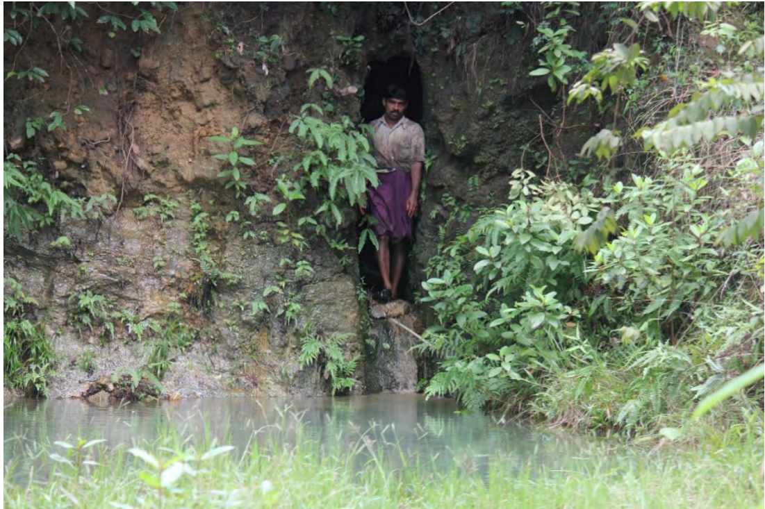
Figure 5.45: A worker coming out from a suranga after completing maintenance.
