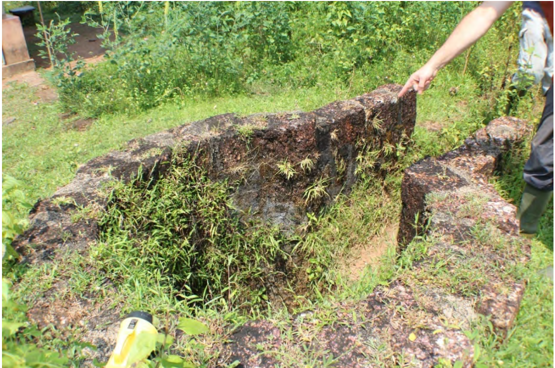
Figure 5.37: An outside view of an airshaft, which opens into a working suranga .
