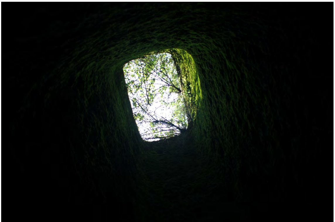
Figure 5.40: View from inside a suranga through an airshaft.
