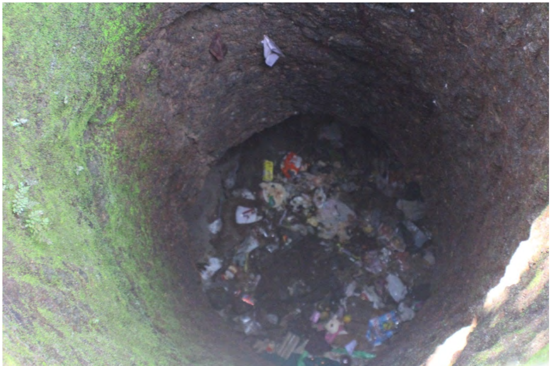
Figure 5.38: Looking down an airshaft in a dry suranga .
