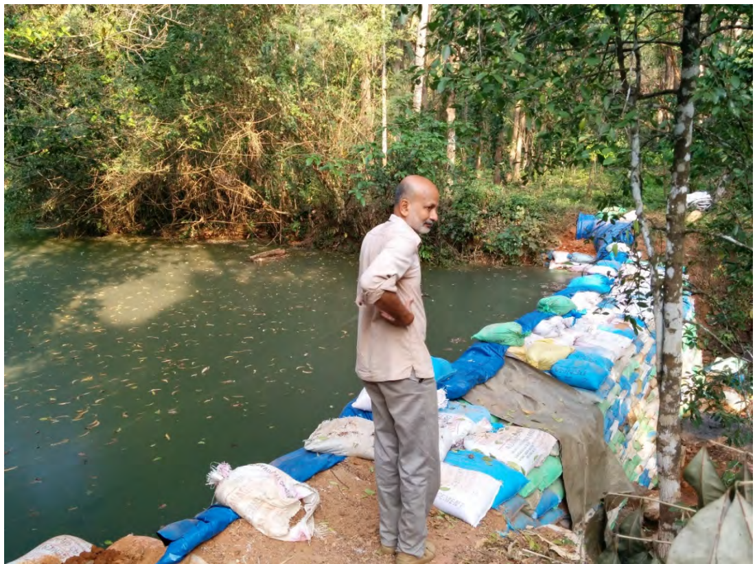
Figure 7.17: A temporary check dam on a seasonal river made by sandbags.
