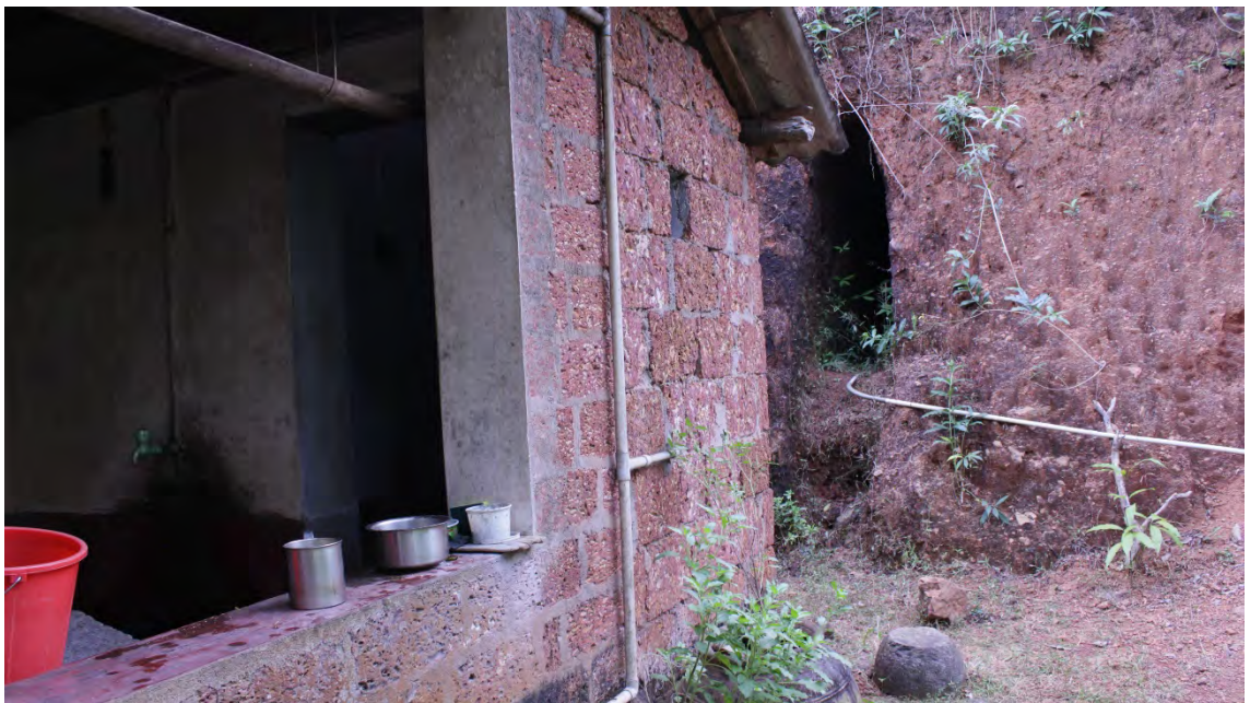
Figure 7.11: An elevated suranga excavated into a hill slope in the backyard of a house.
