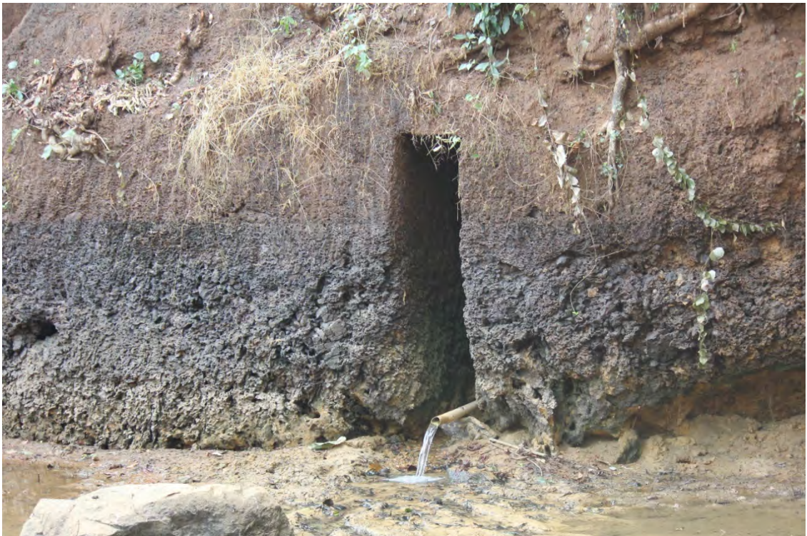
Figure 6.3: A suranga with exposed, black, permeable, hard ferricrete layer.
