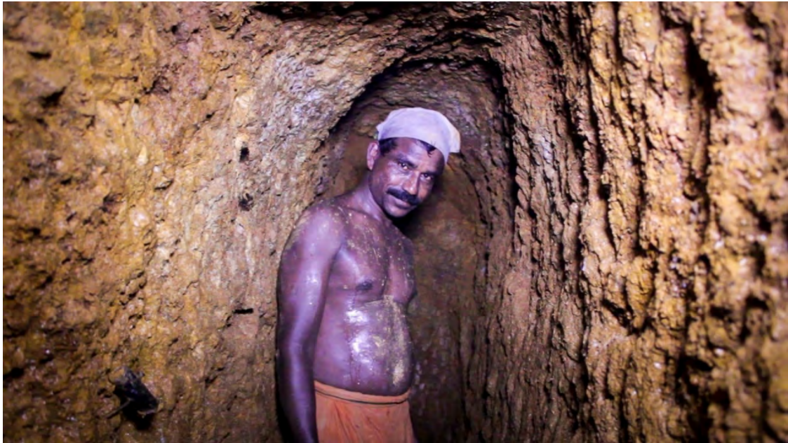
Figure 5.3: Inside view of a typical suranga tunnel, during excavation of a suranga .
