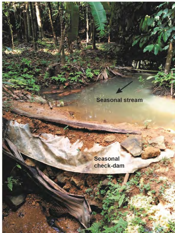
Figure 7.16: A temporary check dam made of soil and rocks on a seasonal stream.
