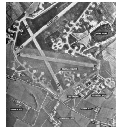
15. Redundant MOD land at Deenthorpe in Northamptonshire
