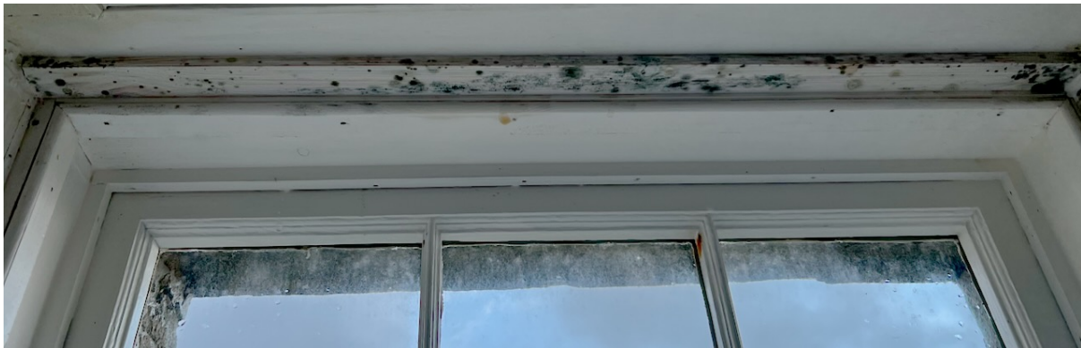
Figure 43: The proliferation of Cladosporium moisture-laden wooden periphery, impervious to pre-emptive application of ostensibly 'mould resistant' commercial paint. Symptoms manifested by individuals exposed to Cladosporium include but are not limited to, headache, fatigue, breathing difficulties, chest pains and inflammation of the eyes. The emergence of this mould signifies water incursion or dampness. (Author's image)
