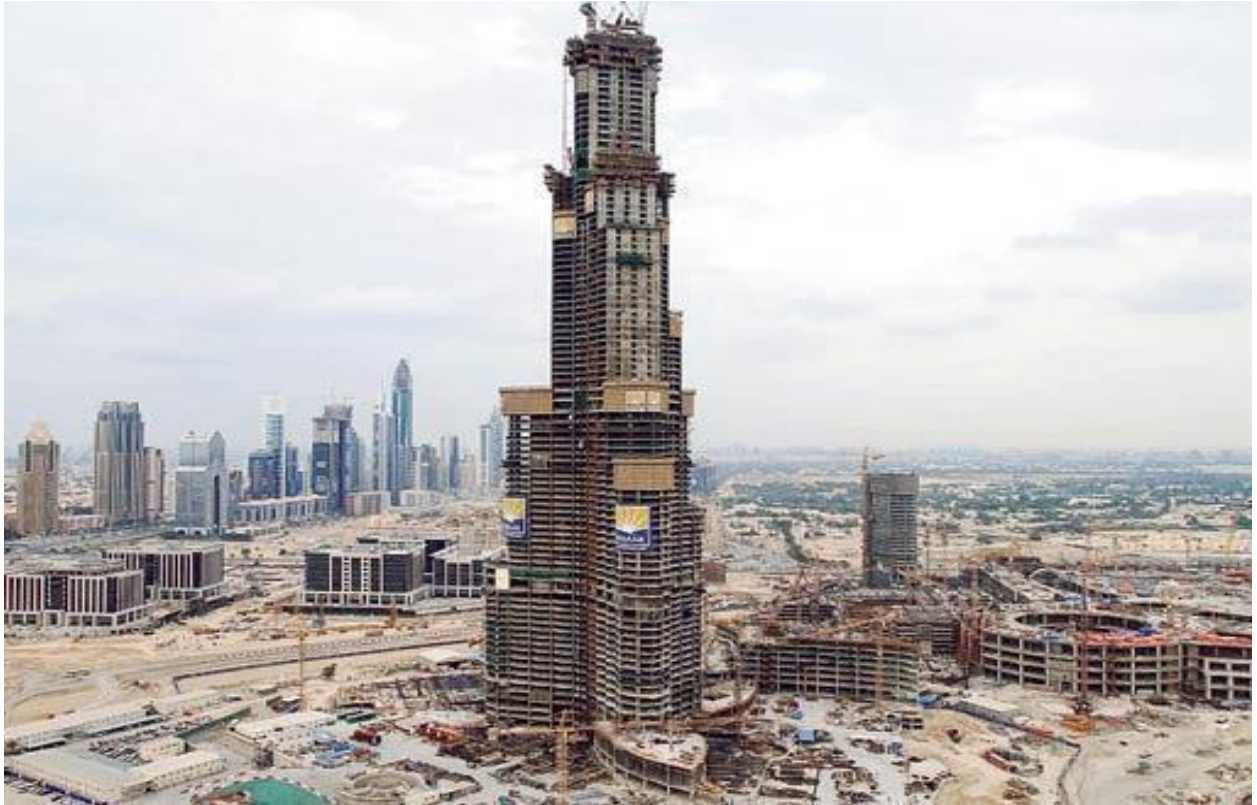
Figure 5-62 Construction stage of the tower (Burj Khalifa Facts and Information, 2023)
