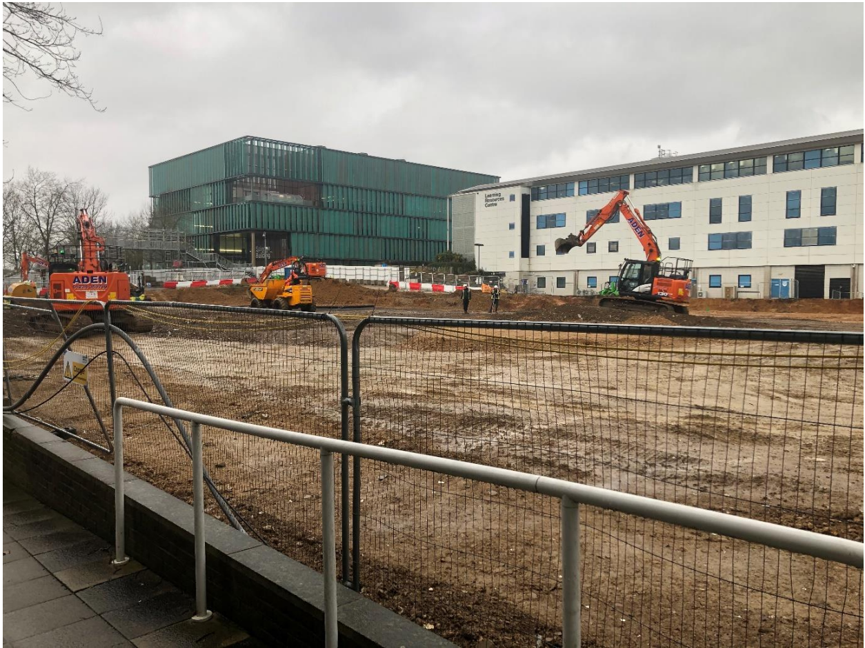
Figure 5-42 Site preparation and levelling the ground
