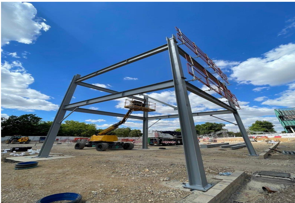
Figure 5-47 Steel columns and beams installation
