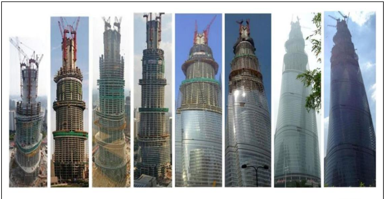
Figure 5-89 Construction stages of Shanghai Tower (Zhang et al., 2016)
