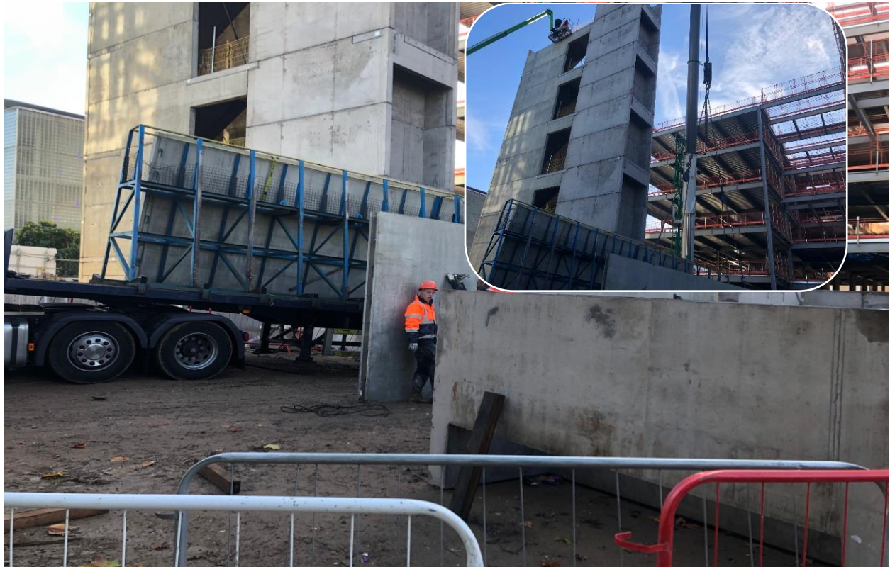
Figure 5-44 Prefabricated concrete transporting
