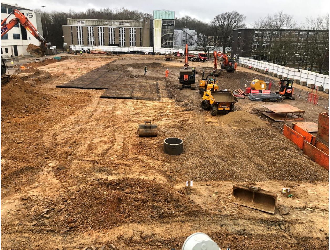
Figure 5-41 Excavation and site preparation
