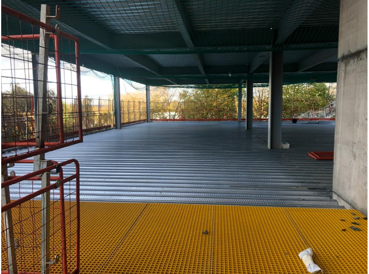
Figure 5-49 Typical floors safety net
