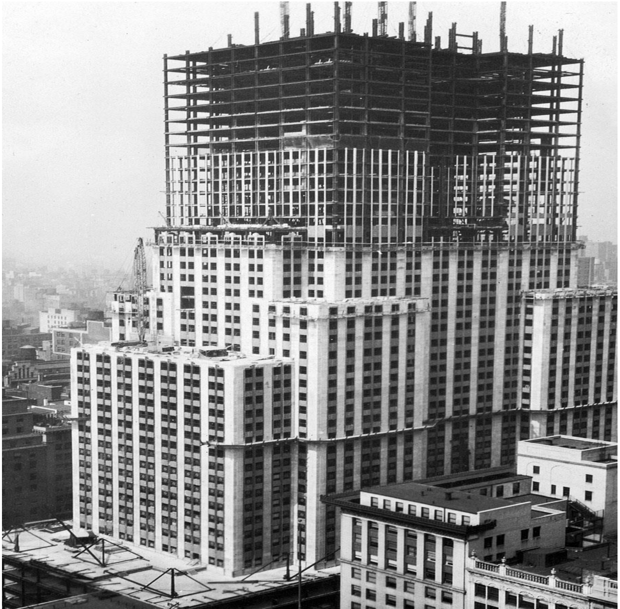
Figure 5-81 Construction of high floors (Geographic Guide, 2022)
