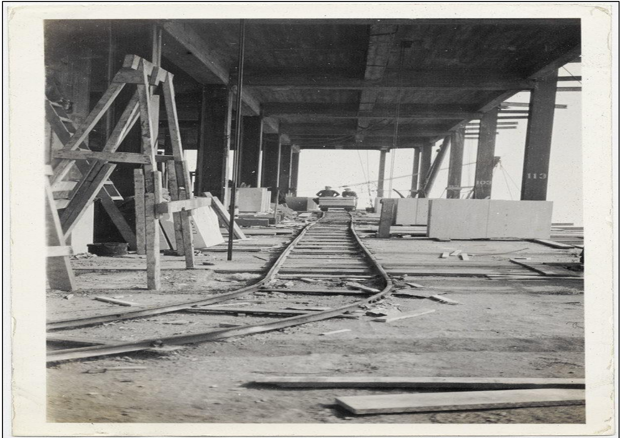
Figure 5-80 Construction works (Jacobsson and Wilson, 2018)
