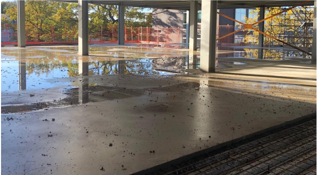
Figure 5-43 Typical floor slab in SPECS Project
