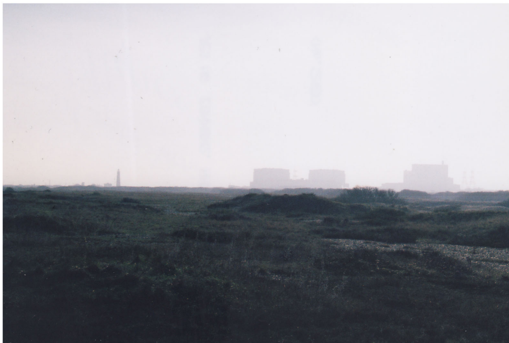
Figure 2. Looking across Denge Marsh to Dungeness power station and lighthouse (photograph by author, 2006).
