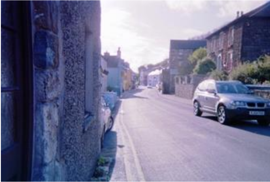
Photograph 13: "House on the corners of the bridge" (L136)
