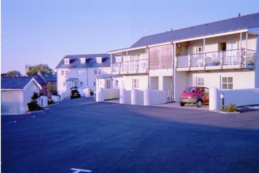
Photograph 25: "St David's, St Non's apartments" (L56)
