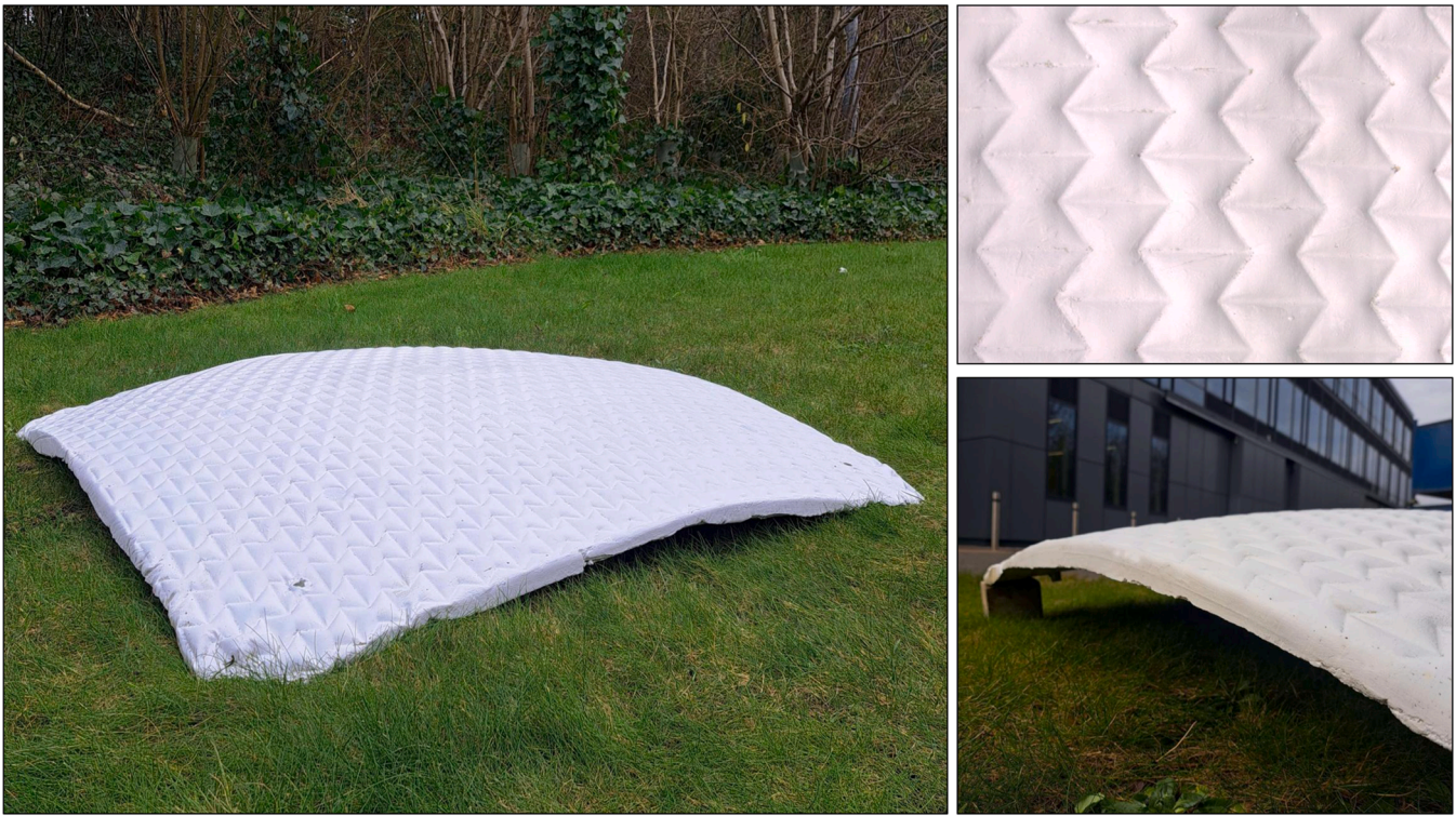
Fig. 11. Concrete shell (Shell 2) cast using an auxetic grid as a formwork.
