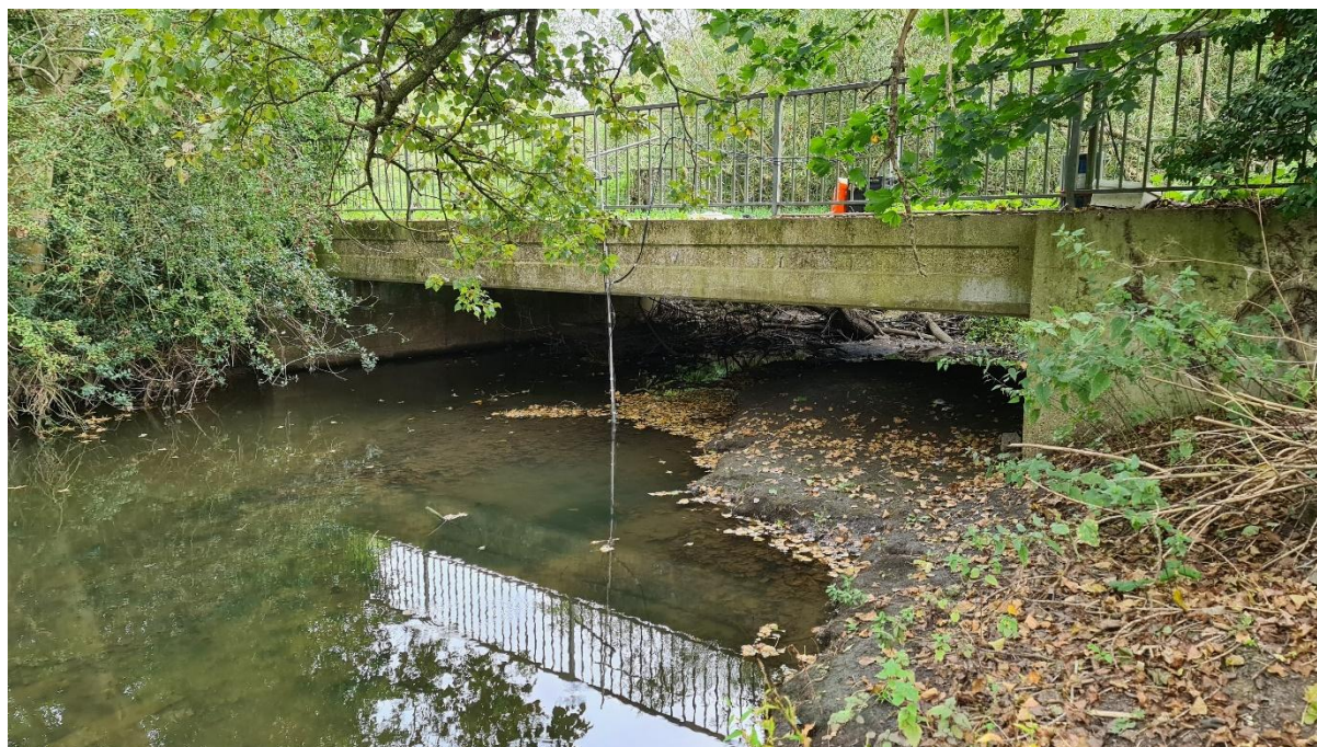
Figure 4. 3: The stage, turbidity, conductivity and water temperature gauge were installed in May 2023 at Drop Lane by affixing an aluminium pole with the probes secured to it to the railings of the Thames Water owned bridge. This is the view looking upstream of the River Colne with the vertical pole of the gauge inserted into the river channel. (27 September 2023).
