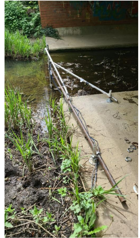
Figure 4. 2: Left: The initial temporary station hammered into the banks of the Colne just before the bridge, with the stage and turbidity sensor attached to it and wired to the box kept within the EA box on the side of the bridge. (25 November 2022).
