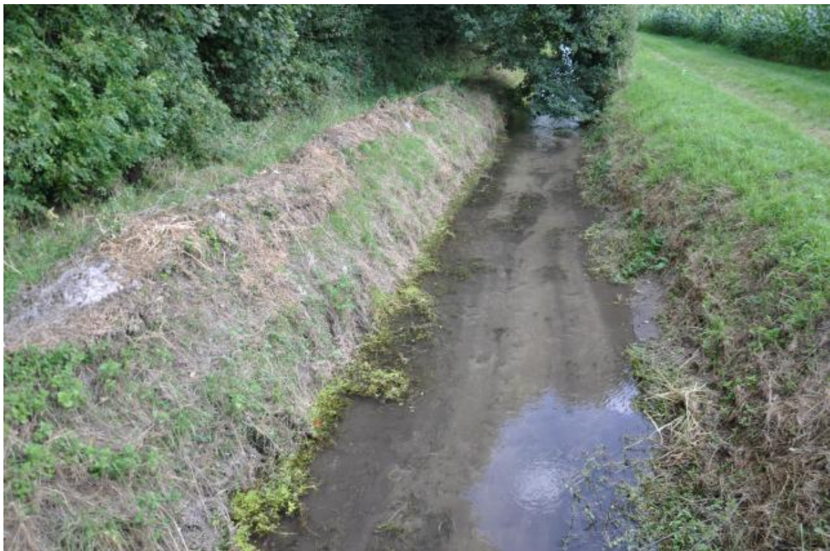
Figure 1. 20: The Gaywood River after vegetation removal on the banks and in-channel (Sennitt, 2023).
